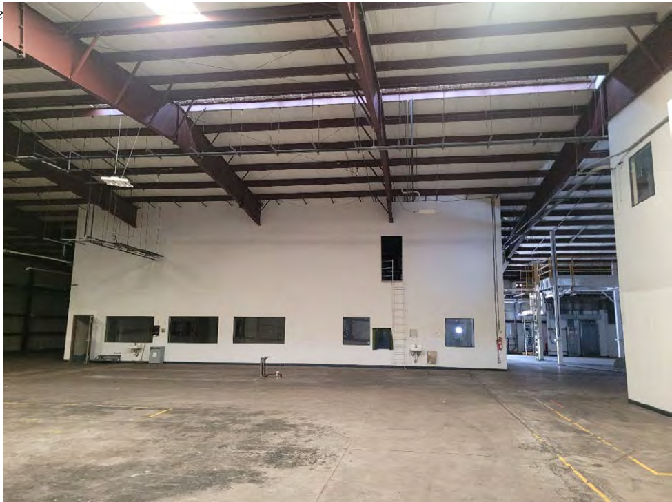
b. View of warehouse interior.
