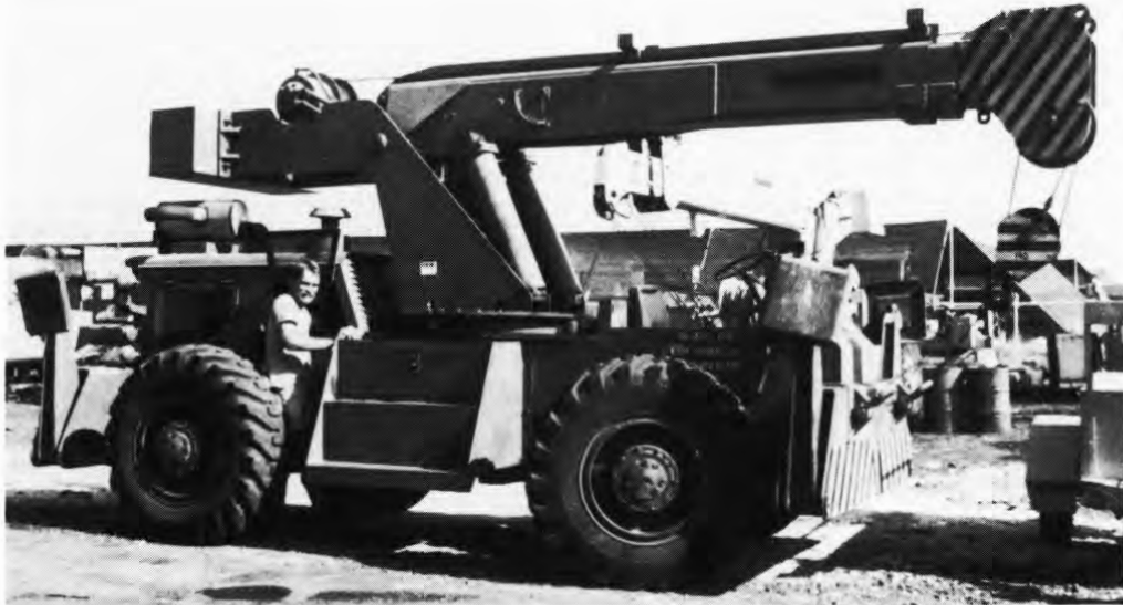
Steve Wilson is dwarfed by the 15-ton hydraulic crane used to move machinery, install pumps offshore, lift vehicles and other heavy-duty tasks at the NELH Kona Seacoast Facility at Keahole Point, Kona.
