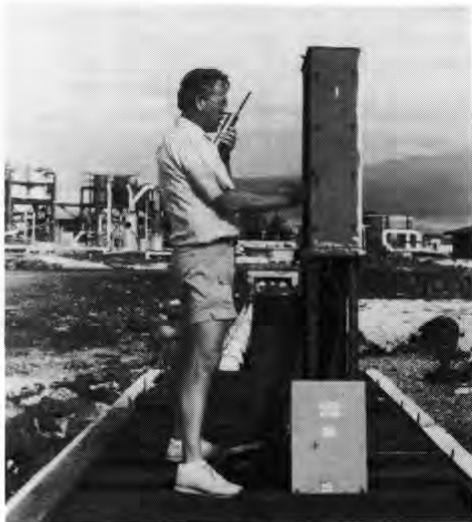
Underwater electrical cable installation is remotely directed by Aarne Haas.
