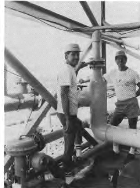
Ernie Galt (left) and Hal Link conduct experimental runs to collect data on open cycle OTEC subsystem components.
