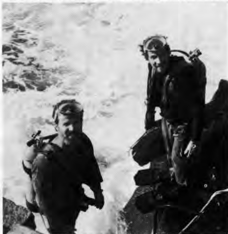
Kent Merrill (left) and Jan War (right) prepare to jump into the foamy brine to secure underwater connections at the offshore pump station.
