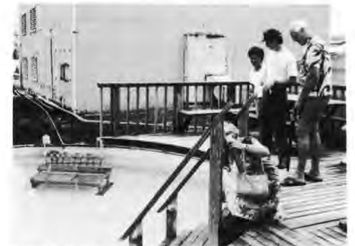
DBED Energy Extension Agent Steve Holmes explains how the PGF demonstration spa is heated with a submerged heat exchanger using geothermal heat.
