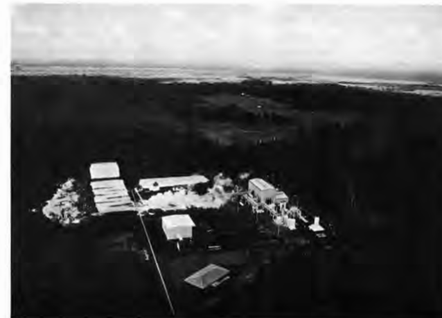
Aerial view of the Puna Geothermal Facility.
