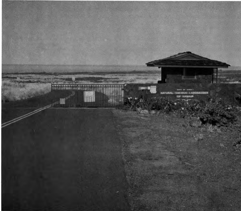
Entrance gate and guardhouse with laboratory in background.
