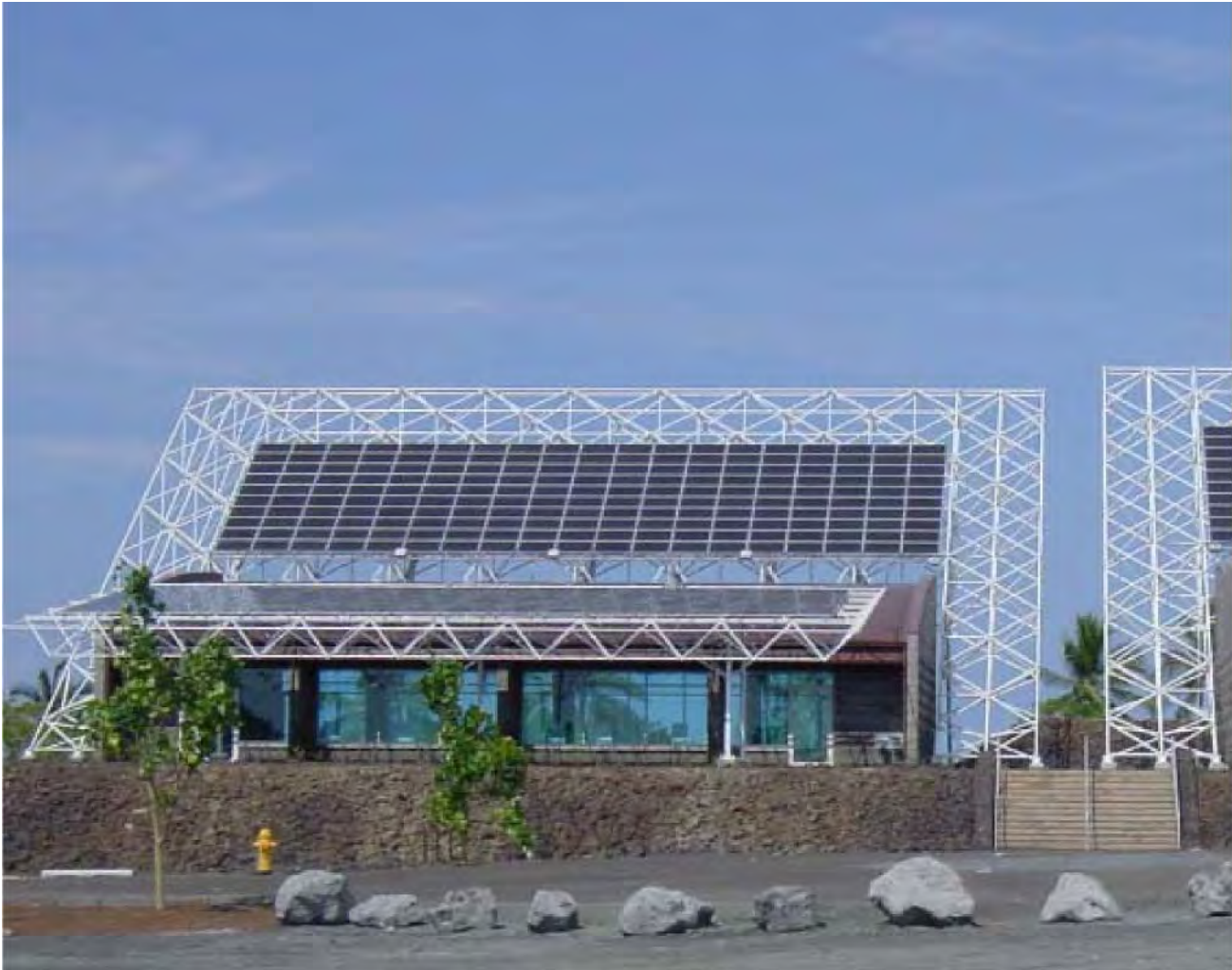
A view from the parking lot of the main building of the new Hawaii Gateway Energy Center at NELHA. Its photovoltaic panels mounted on distinctive "space frames" are owned and managed by the Hawaii Electric Light Company, Inc. and provide power to the grid.
