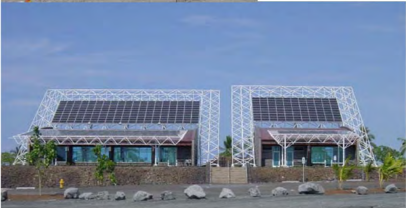
The Hawaii Gateway Energy Center (HGEC) at NELHA is distinguished from afar by the “space frames” that support photovoltaic panels. Passive solar design allows energy-efficient temperature control of these two main buildings, driven by deep seawater cooling.
