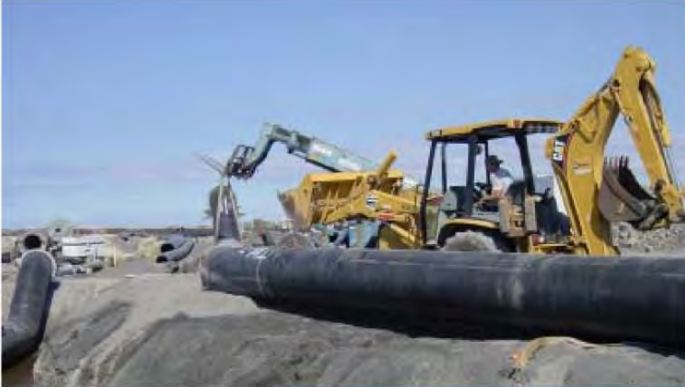
Some views of work on the onshore distribution system for the 55-inch pump station that will service tenants in NEL HA's HOST Park properties:
