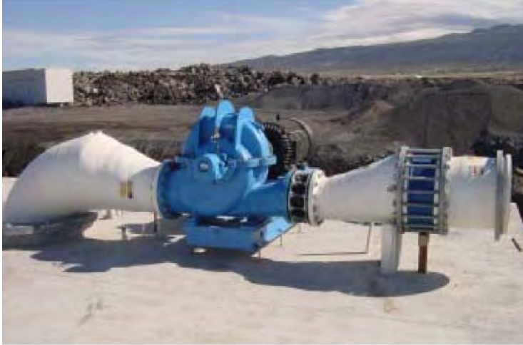
One of the 200 HP Gould split case centrifugal pumps awaiting installation in the surface seawater supply section of the new 55-inch pipeline pump station.
