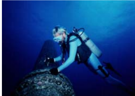
A professional diver works on a pipeline in waters at Keahole Point during early years of NELHA's development
