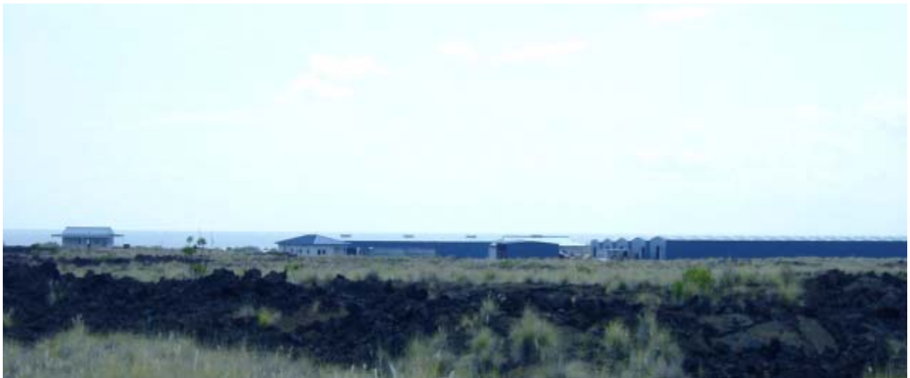
During FY03, NELHA tenant Moana Technologies LLC completed the major portion of construction of distinctive new blue and white research and development buildings at an 11.4 acre site at NELHA. These will house state-of-the-art shrimp broodstock culture facilities.
