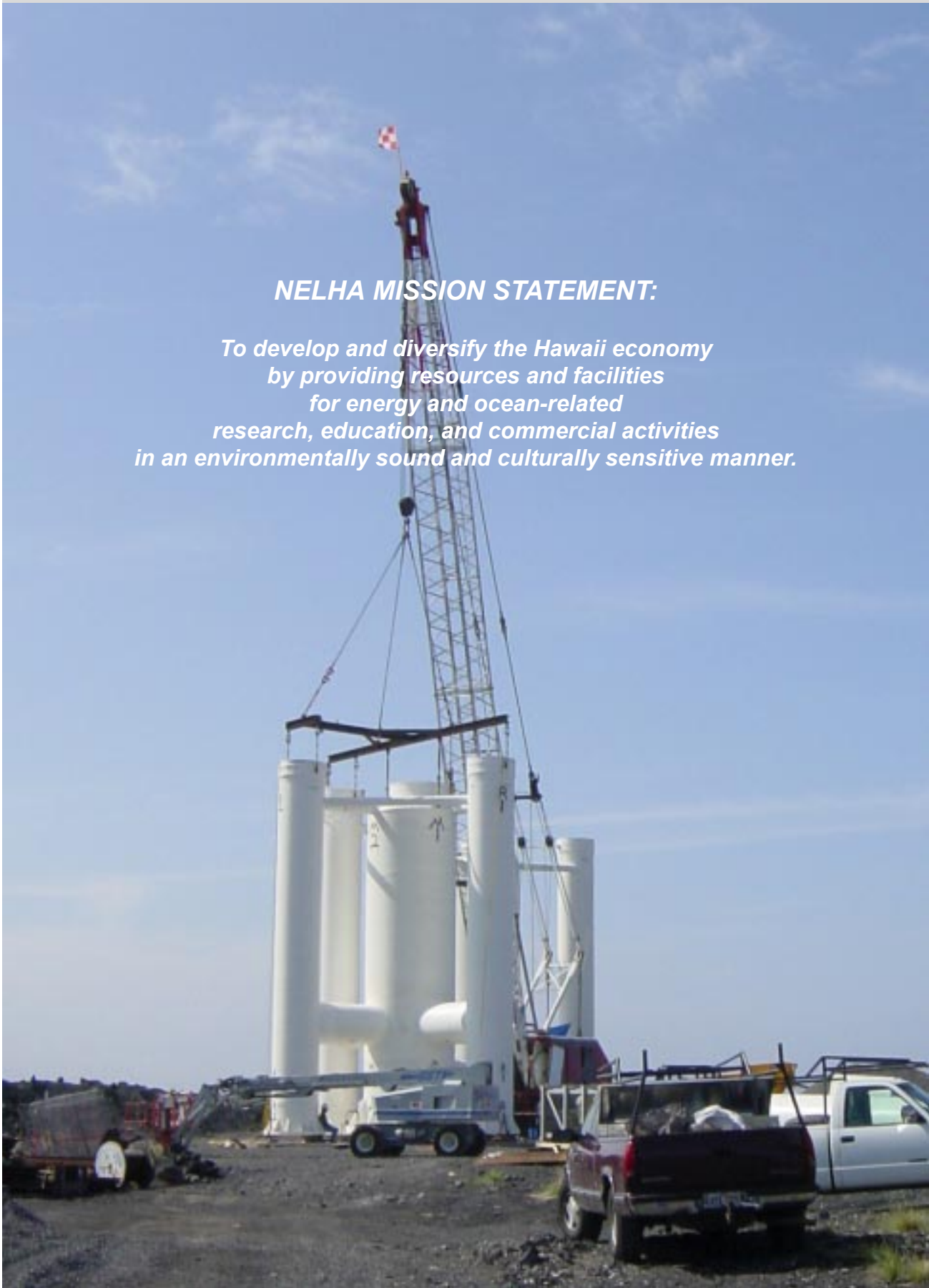
The 40-ft. tall fiberglass-reinforced plastic canister, specially fabricated for the 55-inch pipeline pump station in HOST Park, dominates the work site above the underground sump where they will be installed.
