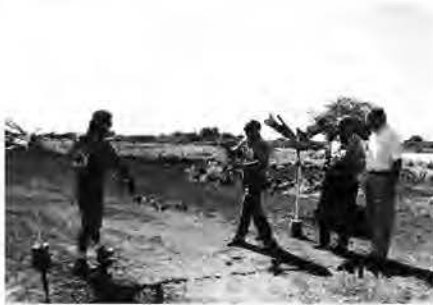
The Board of Directors and NELHA Staff untie the maile at a dedication ceremony for the new Booster Pump Station in October 1998.
