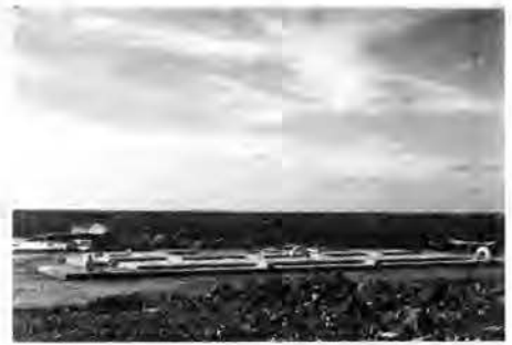
The underground main NELHA pump station at Keahole Point provides warm and cold seawater to all current NELHA tenants.
