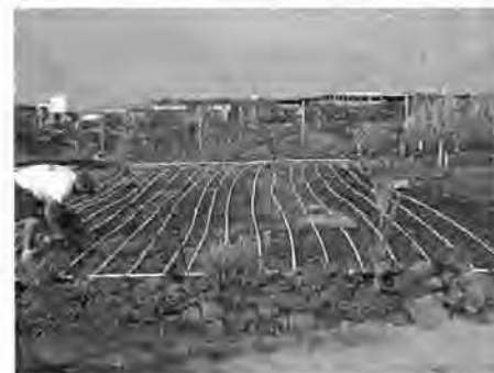
A demonstration site for "eco-turf," proposed for golf courses of the future, is prepared by burying an underground heat exchanger which will chill plant roots with deep seawater.
