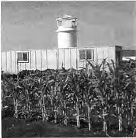
ABOVE: In the background, the CHC "Hurricane Tower" extracts freshwater from seawater, while, in the foreground, deep seawater successively cools the Chillhouse and the roots of a thriving row of corn growing in the organic demonstration garden.
