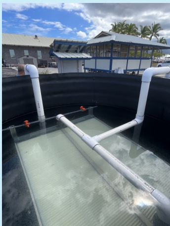
Above: Submerged membranes in Pacific Filtration System demonstration at the NELHA makai research campus. Photo courtesy of PFS.
