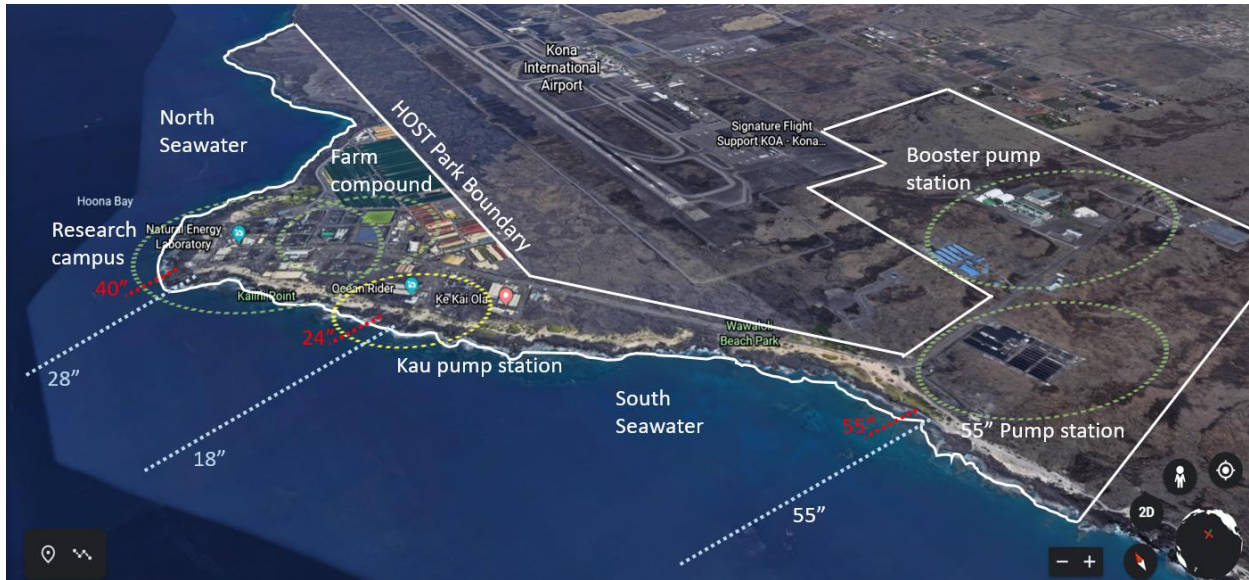
Figure 2. Five major electrical load sections owned and managed by NELHA The image was created using a Google Earth image. The seawater pipes are pictorial representation, not to scale.
