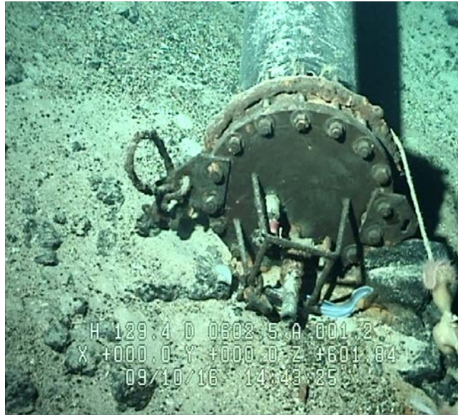
Figure 11 – Blind Flanged Intake of 18D at 602M
