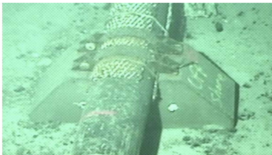
Figure 4 – Example of Concrete Gravity Anchor Attached to 18" Pipeline
