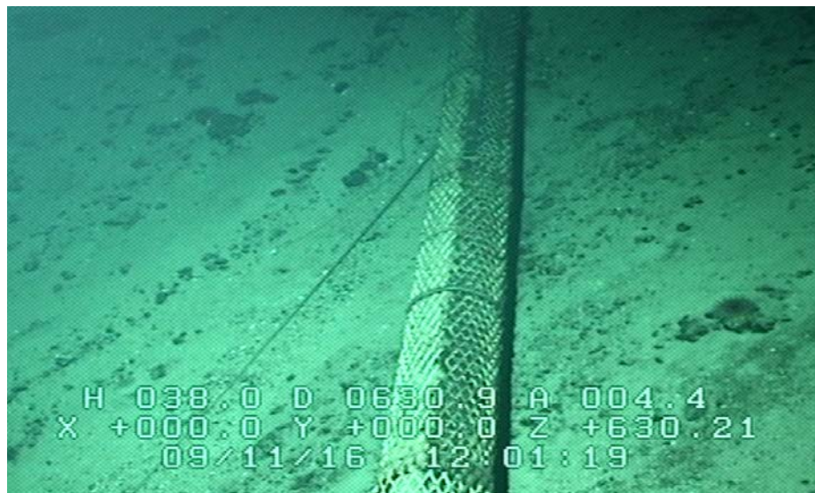
Figure 2 – 18" Ocean Farms of Hawaii Pipeline with Expanded Metal Grating
