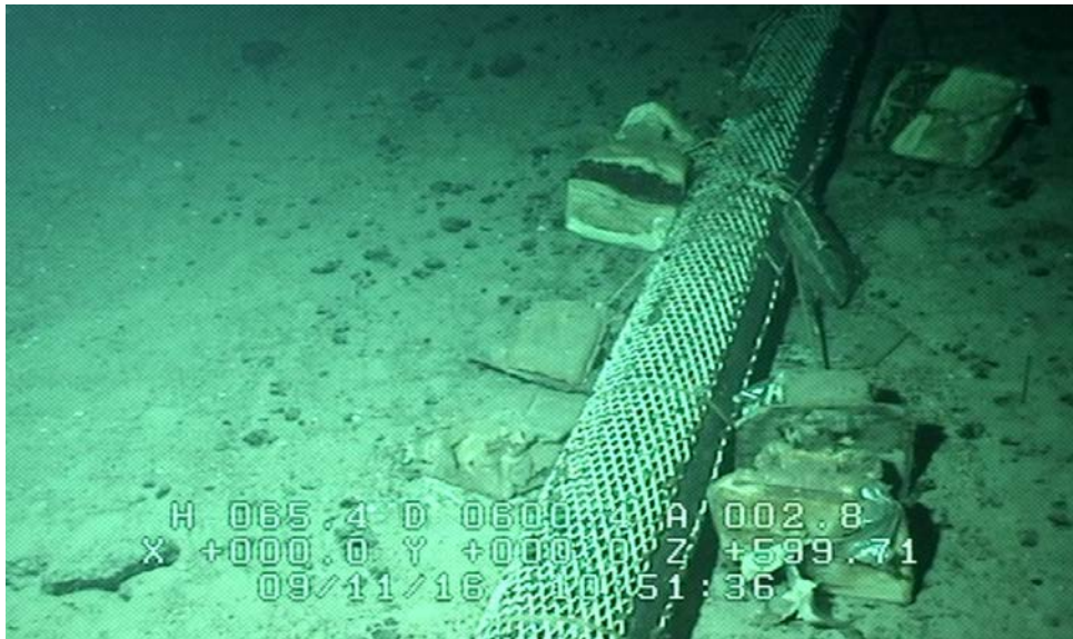
Figure 3 – Crushed Foam Floatation Units still attached to Pipeline
