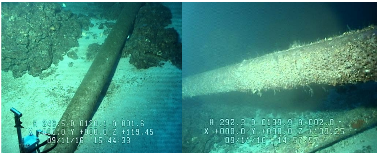
Figure 1 - Sections of Abandoned 15" PVC Pipe on Bottom in Various Locations
