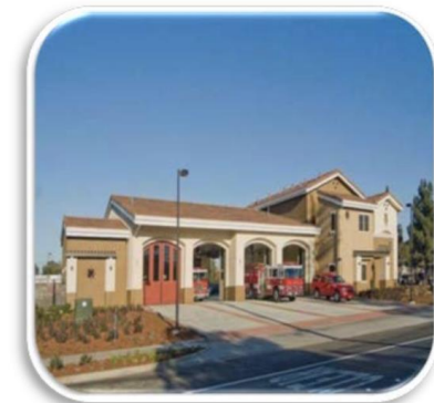
City of Fremont Fire Station
