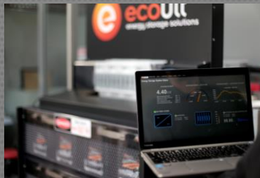
SCADA & CLOUD COMMUNICATIONS
