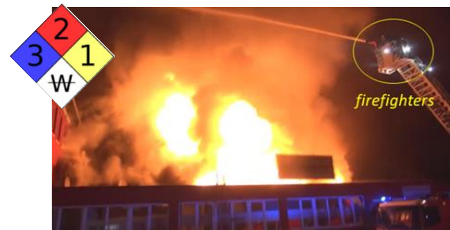
After a fire was contained, this photo captures the initial explosive re-ignition of a 2.5MWh lithium battery, severely injuring 3 experienced firefighters in Hilden, Germany
