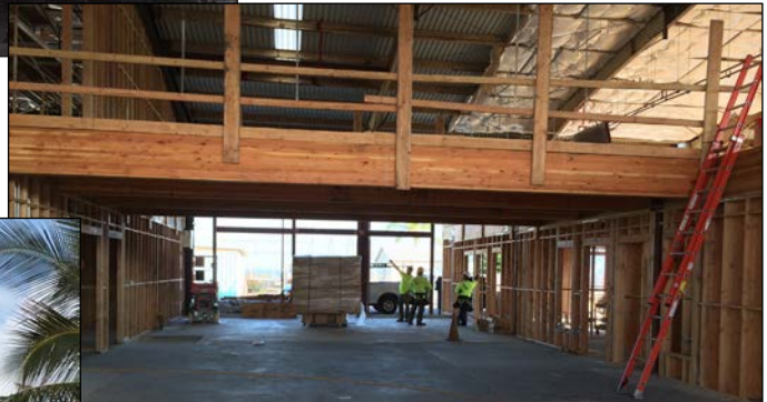
New walls and mezzanine erected
