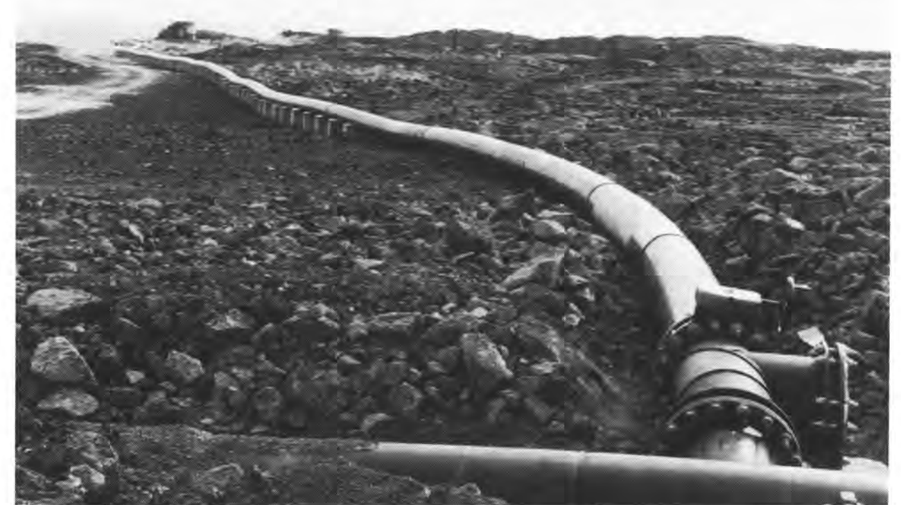
The newly installed 18-inch diameter emergency back-up pipeline snakes across the lava towards the sea. This pipeline will deliver 3000 gpm of deep cold seawater to NELH projects.
