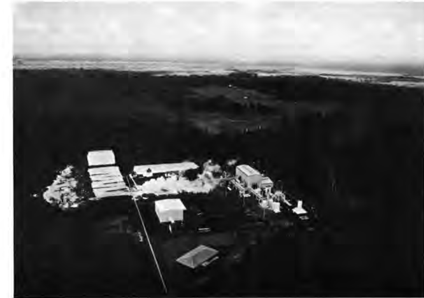
Aerial view of the Puna Geothermal Facility.
