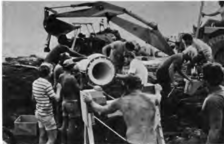
All hands at work on the installation of a Hawaiian Abalone Farms deep seawater pipeline, August 1986.
