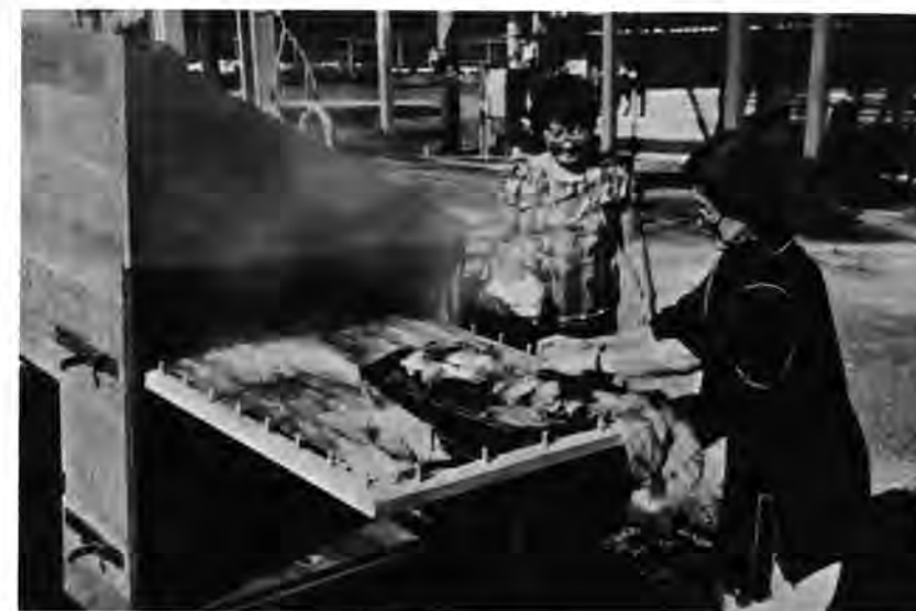
Using geothermal steam to fix dyes in Japanese silks.
