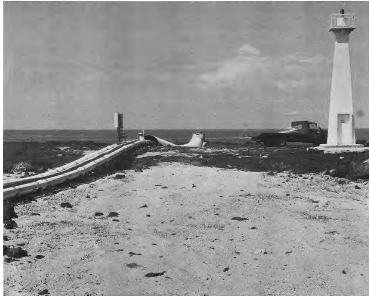
Onshore section of seawater pipelines. Note protective cover extending from the lighthouse to shore.
