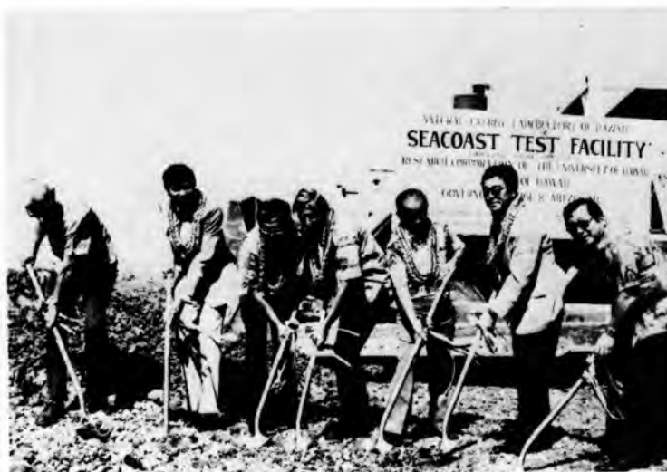
Seacoast Test Facility Groundbreaking
