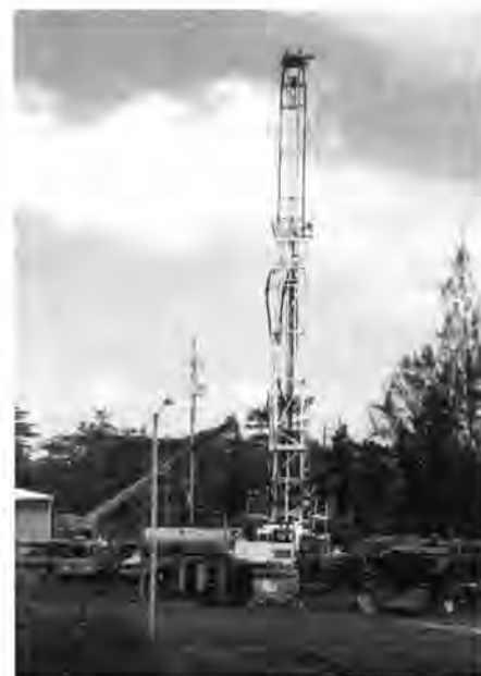
Drill rig looms over the PGF facility site during the plug and abandon procedures for the HGP-A well.
