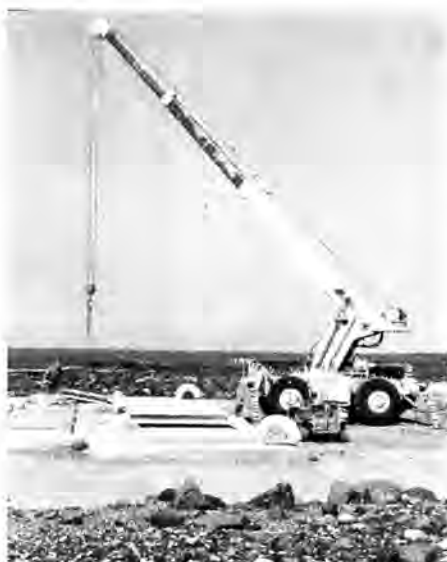
A crane is needed to lift the heavy concrete covers to the NELHA main pump station at Keahole Point.
