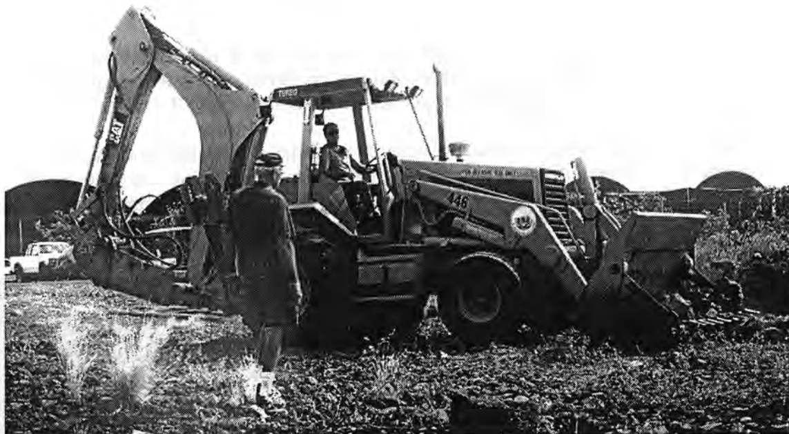
Earth-moving heavy equipment is used in many tasks performed for NELHA tenants as their sites are prepared for occupancy or expansion.
