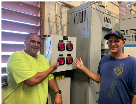
Above: Chad Debina (left) and Kevin Tapley (right) point at research campus electrical meters connected to the NELHA SCADA system.
