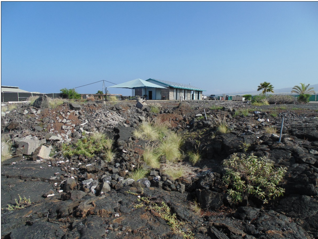
Figure 6. Developed mauka portion of the parcel, view to the north.
