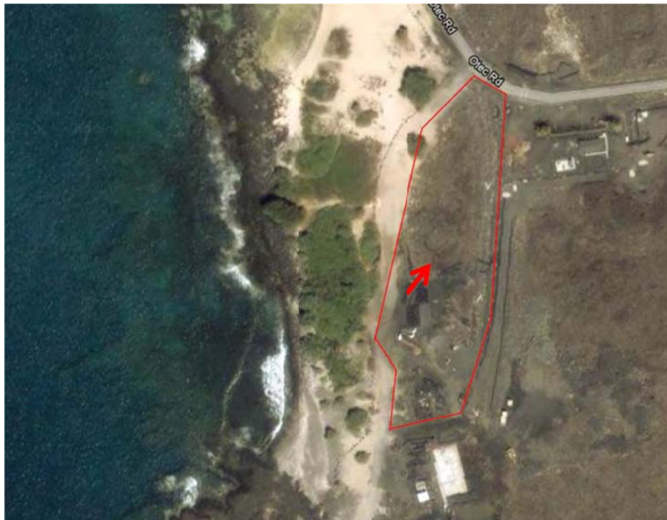
Figure 9. Aerial photo of the 1.76-acre lot allocated for OTI RD&D Facility; NELHA 55-inch Pump Station is south of the OTI lot.
