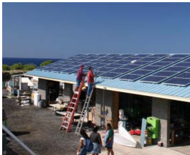
WHEA students and adult colleagues work collaboratively on final stages of installation of new photovoltaic panels at the public charter school's NELHA site.
